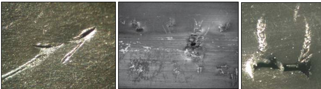
Figure 18. Examples of rodent damage, generally with characteristic scratch marks
