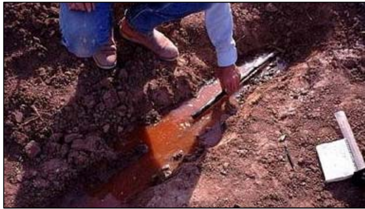
Figure 14. Chemical precipitate flushed from tape. The unidentified chemical compound was supposed to be a fertilizer. It was injected downstream of the filters and plugged a complete irrigation system.
