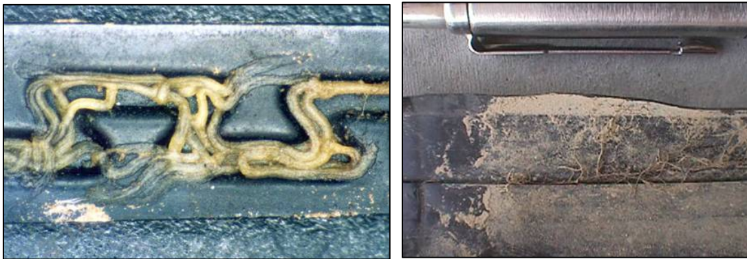
Figure 9. Examples of root intrusion
